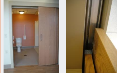
*Variations of surface sliders include bi-pass or "slide-by" doors in renovations and configurations where a wider opening is desired but insufficient wall space is available for stacking when open. Saint Margaret's, New Orleans, 2015, Blich+Knevel.
