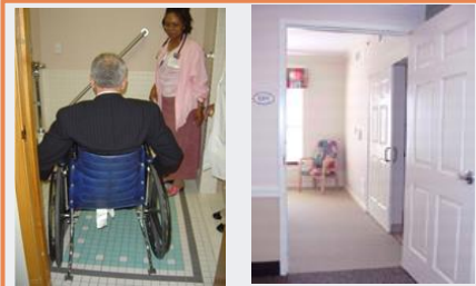
Left: Door widths of 42+'' clear allow staff to push from behind and moved past and around the wheelchair for positioning the next transfer procedures. AFRH, Post Occupancy Study. Right: Village Shalom, Kansas City, KS, Nelson+Tremain, 1998
